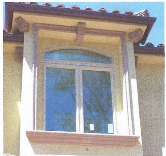
EXAMPLES OF WINDOW SURROUNDS: PFT125S WINDOW TRIM ALONE (TOP) AND WITH PFS518S SILL
